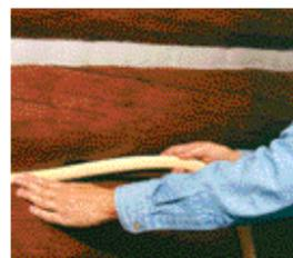
2. Or, install backer rod into caulk well of clean, stained logs.
