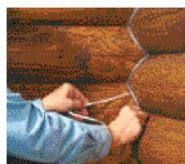
1. Install backer rod into corners of clean, stained logs.
