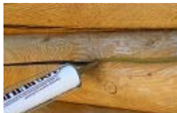
Fill checks and cracks.
