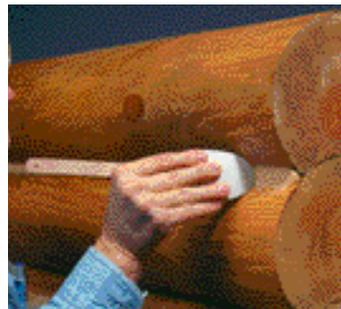
2. Tool to ensure a tight seal to the top and bottom of the caulk line leaving at least 1/4" of caulk in the center of the joint.\*
