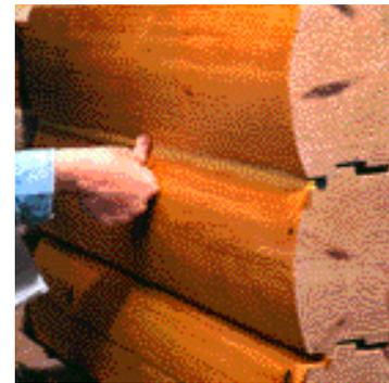
3. Tool to ensure a tight seal to top and bottom of caulk line.
